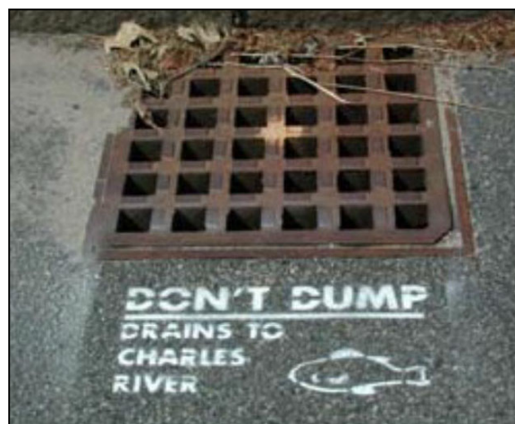
Figure 1: Storm Drain Marking
