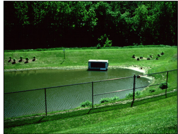
Figure 1: Wet Storm Water Pond
