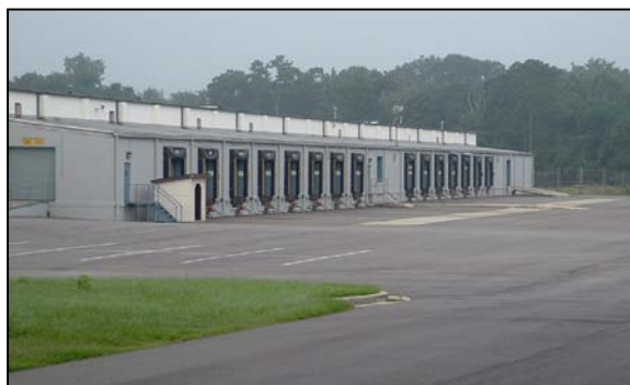
Figure 1: Loading/Unloading Area of Warehouse
