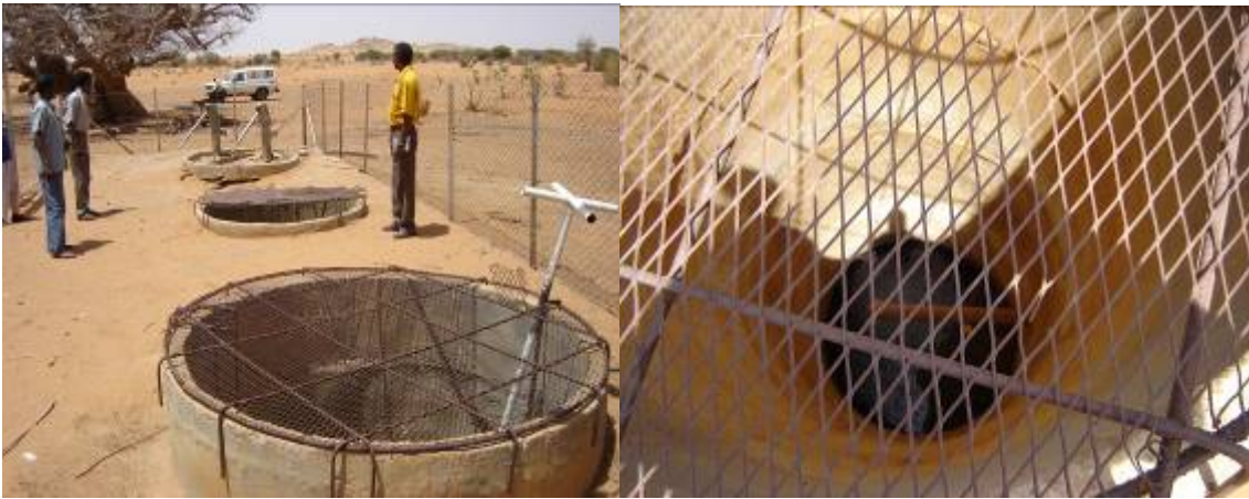
Figure 1. Hafir attached to series of wells, North Kordofan State.
