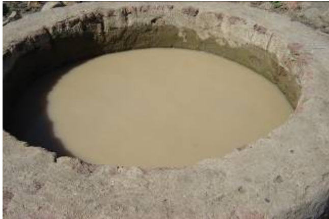
Figure 9: Very turbid water in the abstraction well of a hafir
