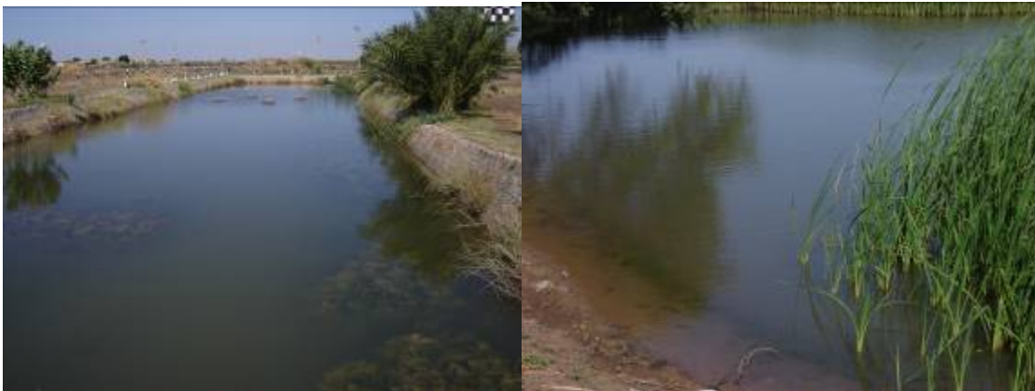
Figure 3. Hafir in Kassala State utilized as a pre-treatment component before slow sand filtration
