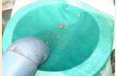
Picture (3.1) coarse filtration screens
