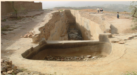
Picture (1.6) Rainwater harvesting Aljerroof
