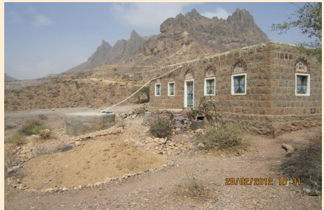
Picture (8.9) Roof rain water harvesting at a house in the village in Yemen [20]
