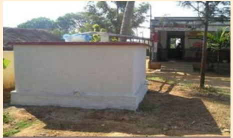
Picture (2.2) Water harvesting tank halfway above ground
