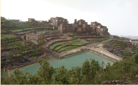
Picture (1.2a) Rainwater harvesting from mountain slope
