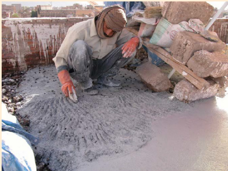
Picture (8.10) Beating the first layer of qadad into the gravel [19]
