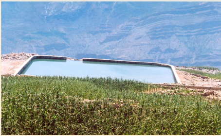
Picture (1.2b) Rainwater harvesting from mountain slope
