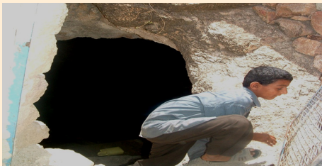
Picture (1.7) Kahf for underground rainwater harvesting
