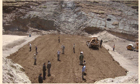
Picture (1.3) Natural foundation for Karef water harvesting
