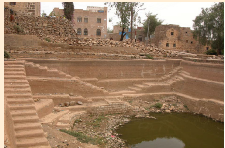
Picture (8.4a) Typical village cistern with Qadad plastering
