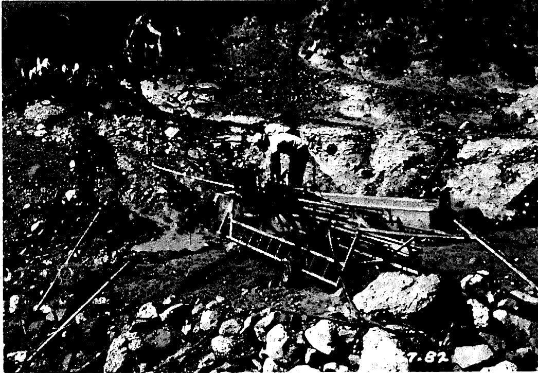
FIGURE 38 Drilling a horizontal well. A standard well casing is drilled on a slight downward slope. Equipment is light and portable and easily transported even in remote, rough terrain. (W. T. Welchert)
