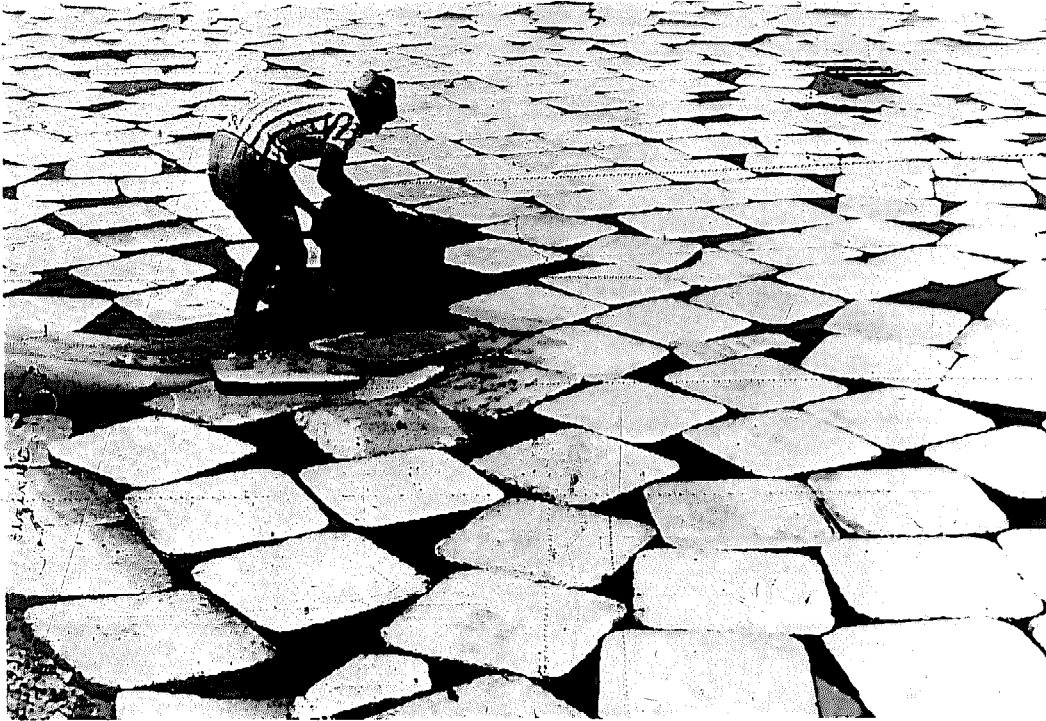
FIGURE 42 Protective covering of molded, lightweight, concrete slabs cut evaporation by an estimated 80 percent recently in full-scale tests on two reservoirs in Ovamboland, South-West Africa. Engineers cover reservoirs with 24-in 2 , 2-in thick floating slabs of polystyrene, sand, and concrete. Exposed surface of each slab is painted white to reflect the intense sun rays, which hasten evaporation.
