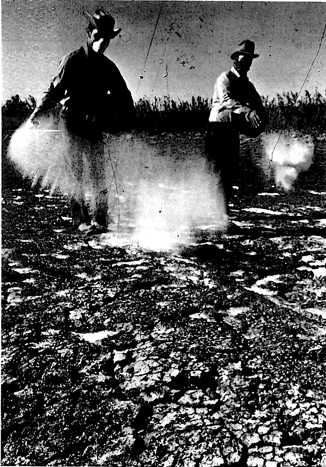
FIGURE 46 Cracked soil structure indicates high calcium content in a dry pond bed in Coconino National Forest, Arizona, USA. Water seeps away through the cracks; original seepage loss in this 1,000 m 2 stock-watering pond was 5-12 cm per day. The dry pond was cleared of rocks and weeds and 1 ton (about US$80 worth) of sodium carbonate applied by hand. This was then mixed with the soil to a depth of about 8 cm, with a small tractor and disk, and . . .
