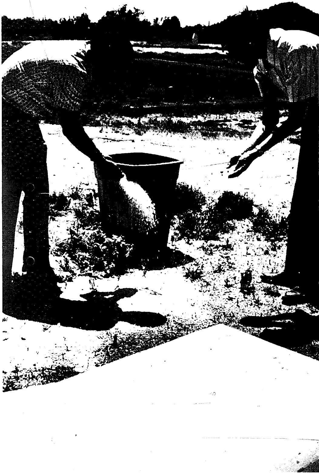
FIGURE 8 Paraffin wax is shredded and spread for rainwater harvesting in Arizona, USA. Melted by the sun, the wax flows into and seals soil pores, making a water-repellent surface that sheds water efficiently. (U.S. Department of Agriculture)
