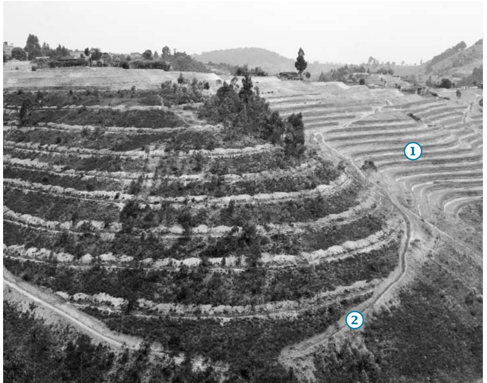
Modified bench terraces and connected waterways, Rwanda
