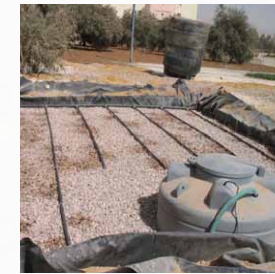
Constructin grey water reuse application at student dormitory
