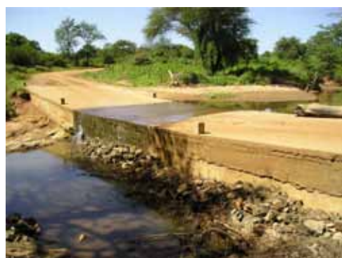
Figure 3: Irish bridge (Source: Nissen-Petersen, E, 2006)
